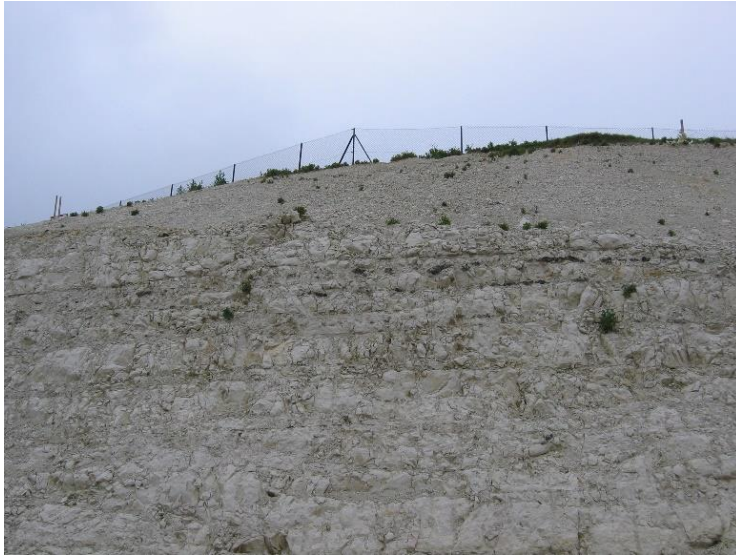
Figure 8: New Pit marly chalk exposed in the temporary cutting for the Weston tunnel, Baldock bypass (TL259339). Note lack of flints common marl seams and common minor joints.
